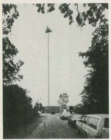
FIG. 1—CELL-SITE BUILDING is dwarfed by the 150-foot antenna tower. The two antennas below the platform are used for reception; the antenna above the platform is used for transmission.
